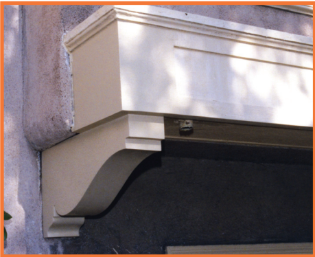
Bracket repair painted and complete.
